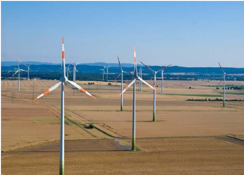
Wind Power Plant.
